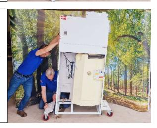
Step 7 Unlock wheels and move to final location
