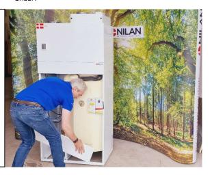
Step 2 Screw in feet to maximise gripping effect
