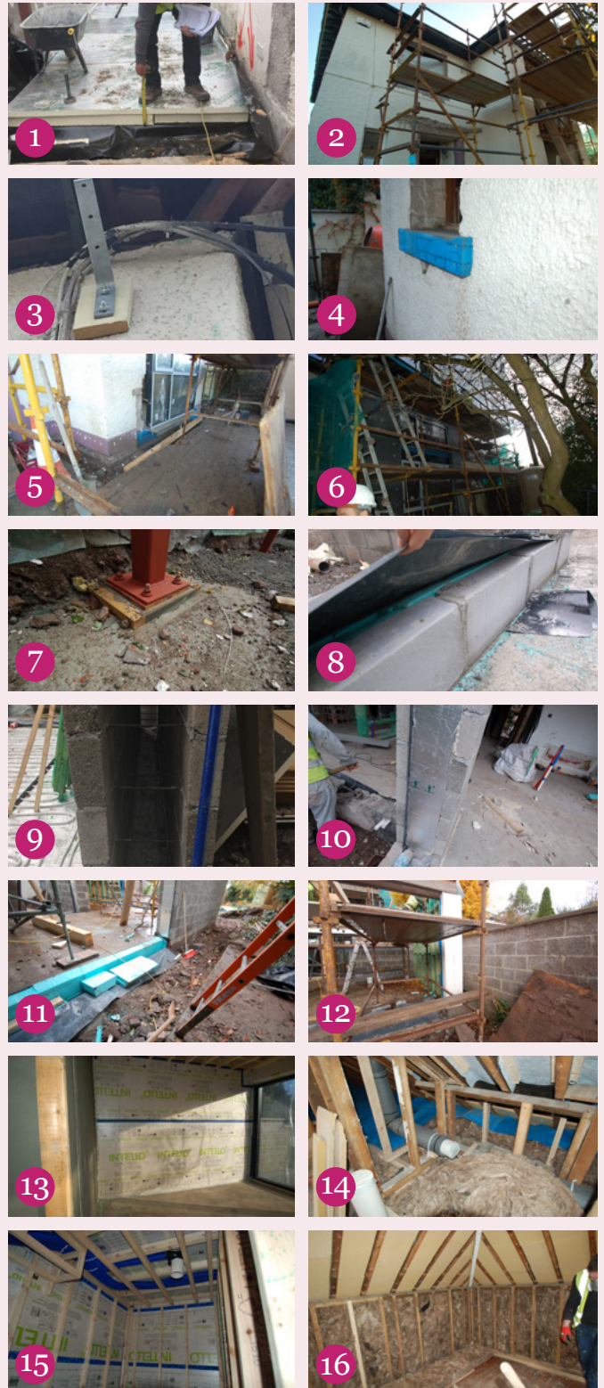
1 150 mm PIR insulation under slab; 2 existing windows removed from front façade; 3 Bosig to electrical brackets; 4 treated timber support wrapped in breather membrane; 5 windows bracketed proud of the walls, to sit in the new external insulation layer; 6 200 mm EPS external insulation fitted to existing front wall; 7 thermal break plate under steel column; 8 Mannok blocks and XPS insulation below DPC; 9 Ancon TeploTies within wall cavity; 10 PIR at window reveals; 11 XPS insulation under threshold to sliders; 12 the timber frame extension wall; 13 Intello membrane fitted to wall and ceiling; 14 insulated MVHR duct in the cold roof space, with ductwork sealed during construction; 15 battens to create a service void inside the airtight later for ductwork; 16 370 mm mineral wool between studs and 22mm Gutex Multitop between rafters.
